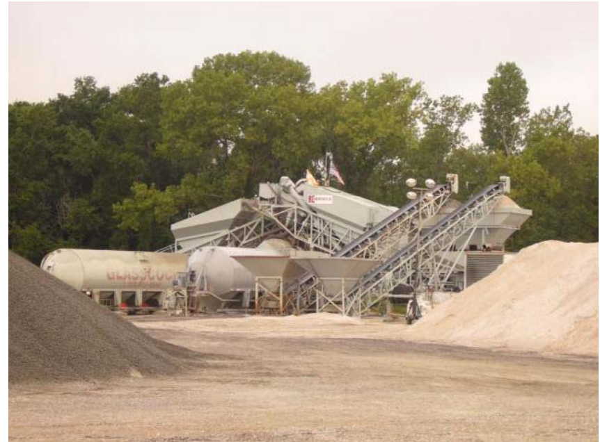
Repair Runway 03/21 RC Construction Batch Plant
