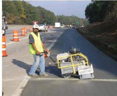
Within the first two hours of placement, an early entry (Soff-Cut) saw cuts contraction joints to match the adjacent mainline pavement.
