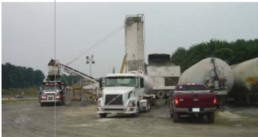
The RCC material is being manufactured on-site in a continuous pug-mill operation. This unit, an Aran ASR280B, produces RCC at rates of up to 500 tons per hour.
