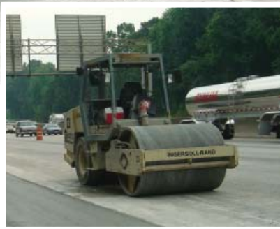
Above & Right: After placement, the RCC was immediately rolled to 98-percent density. Here, a Hamm roller – one of two rollers used on the project – compacts the RCC.
